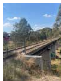
B3.2: Loddon River Bridge
