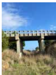
B4.4: Moolort-Baringhup Road Overpass
