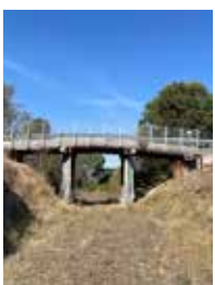
B1.1: Lawrence St Overpass
