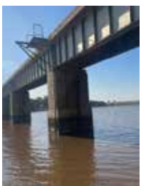
B4.3: Joyces Creek Railway Bridge
