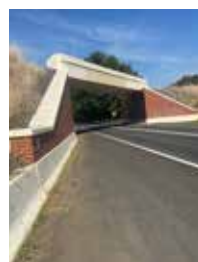
B3.1: Midland Highway Bridge
